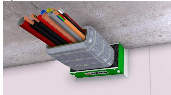
Fig. 6 – Insulate services if required
