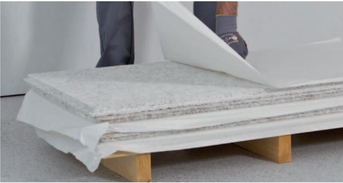
Carefully remove the separating paper layer from the panels and dispose of it immediately. Dust lying on it must not fall onto the panel below.
