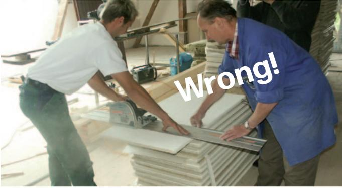
**Not this way!** - Never cut acoustic panels on a stack.
