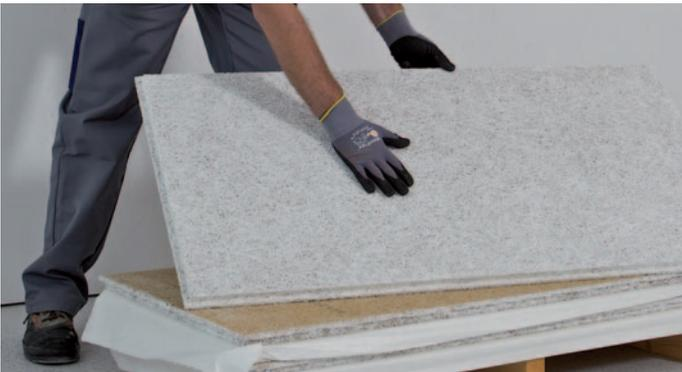
Check panel for damages. Remove any remaining dust with a soft brush.
