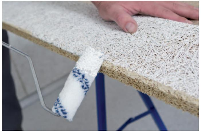
**Painting the bevel** - Use a brush or a thin paint roller to apply the paint.
