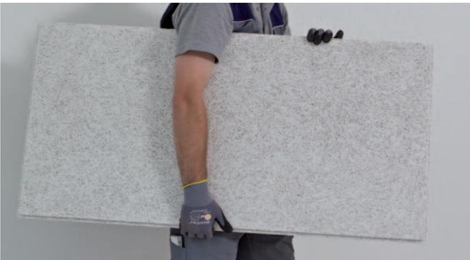
When lifting the acoustic panels from the stack, only carry them on edge. When lifting panels from the stack, never drag them over the edge of the stack in order to prevent damage to the visual side.
