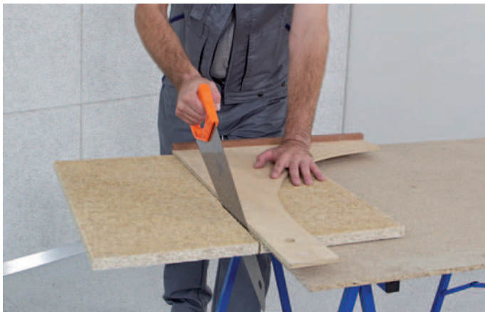
Jack saw – Lay the acoustic panel down with the exposed side up. Always work with a guide. Support the free end of the panel.
