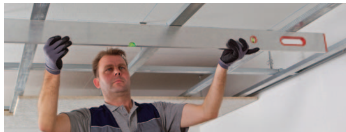
Aligning the Grid with a spirit level or laser level.
