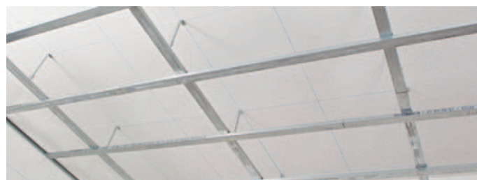
Finished ceiling grid.
