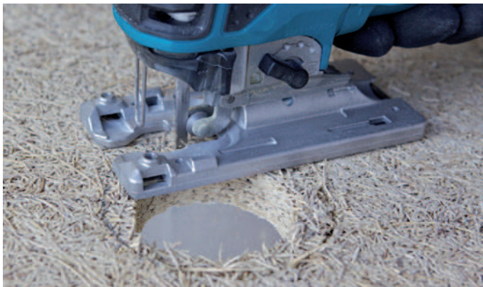
Jigsaw – Lay the acoustic panel down with the exposed side down. Always make longitudinal cuts with a guide.
