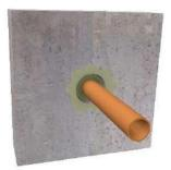
5. Cut nozzle to required bead size and apply sealant around the service and fill the void to the surface
