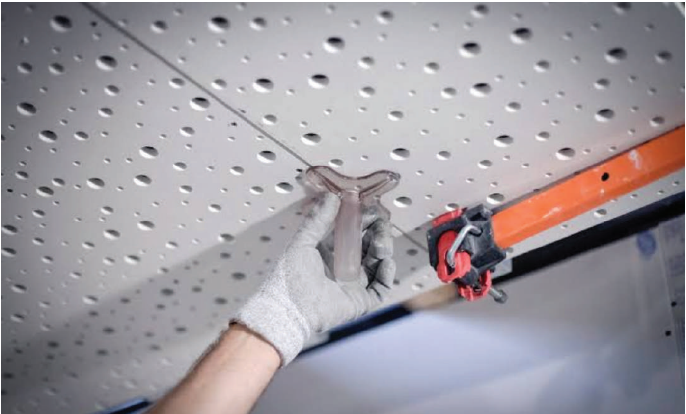
Figure 12: Rigitone Pattern Spacer Tool
