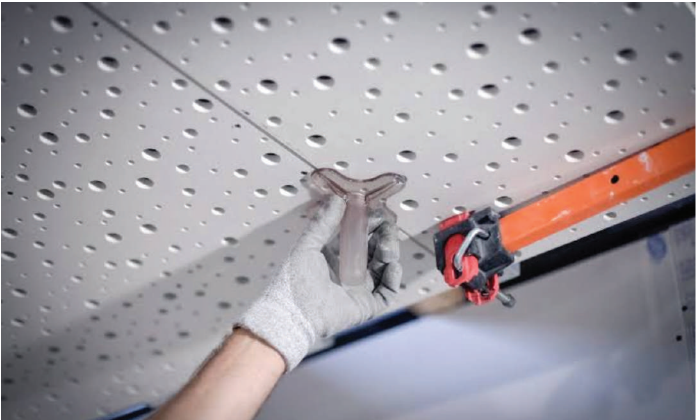
Figure 12: Rigitone Pattern Spacer Tool
