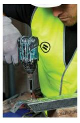
**5/** Attach 45° top connector to cut stud.
