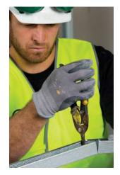
3/ Cut your vertical steel stud to length. Will need to repeat for the two 45° steel studs as per plenum chart provided.
