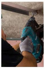
**8/** Drill clearance holes into structure over.
