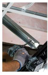
**8/** Connect bracing material to TRACKLOK® fly brace with #10-gauge wafer tek screws.
