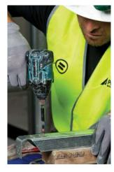
**4/** Attach vertical top connector to cut stud.
