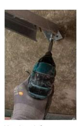
**9/** Fix GRIDLOK® top connectors to structure over with approved anchors.
