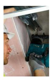
**9/** Drill clearance hole into structure over.
