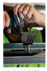
**4/** For TRACKLOK® RETRO screw directly into head track.
