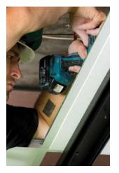
2/ Create 30mm to 40mm clearance hole in ceiling tile with holesaw (pilot bit marks centre point on head track).
