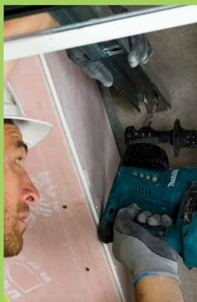
9/ Drill clearance hole into structure over.
