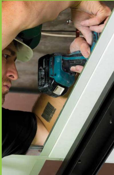
2/ Create 30mm to 40mm clearance hole in ceiling tile with holesaw (pilot bit marks centre point on head track).
