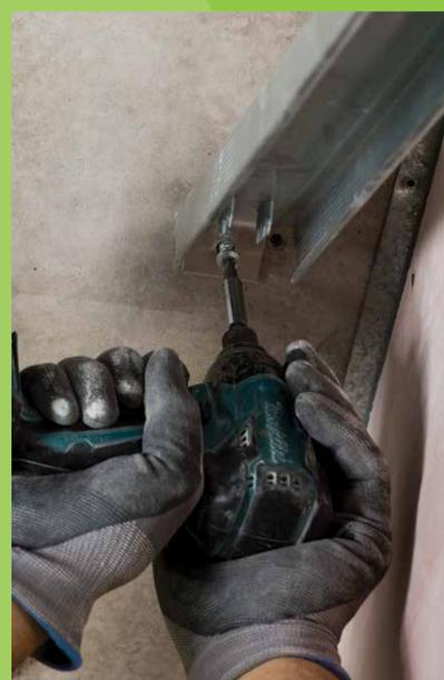
10/ Fix TRACKLOK® top connectors to structure over with approved anchors.
