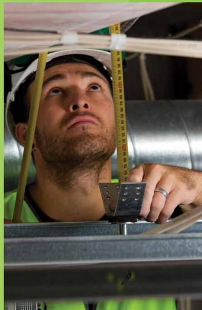
5/ Measure distance to structure from fly plate below screw holes.
