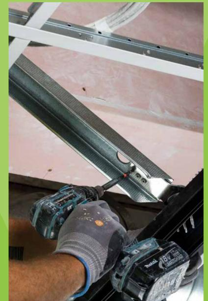
8/ Connect bracing material to TRACKLOK® fly brace with #10-gauge wafer tek screws.
