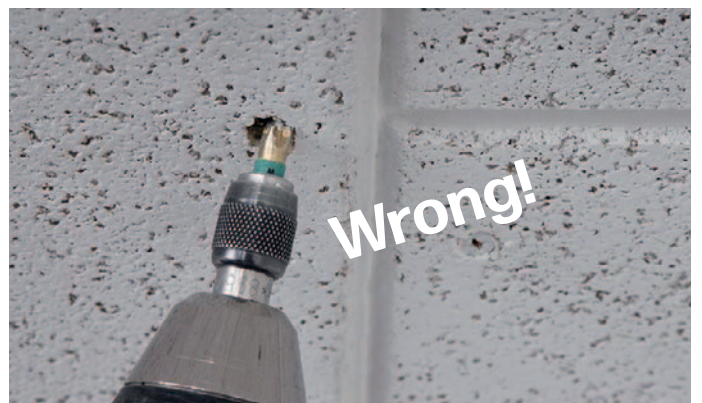
Not this way! - The screw head must be flush with the surface of the panel. A depth gauge should be used to prevent the over-driving of screws into the face of the panel.
