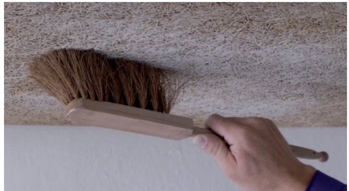
Brushing - Efflorescence, dust, etc. can be removed with a soft brush. Set loose fibres with a commercial grade acrylic primer.
