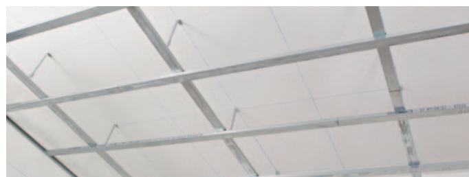
Finished ceiling grid.
