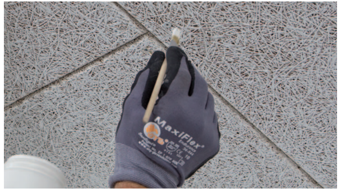
Painting over the screw heads - Use a fine brush to cover unpainted screw heads with the colour of the panels after installation. It is absolutely necessary to avoid double painting of the panel surface around the screw head. This would cause irritating colour differences.
