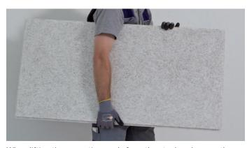
When lifting the acoustic panels from the stack, only carry them on edge. When lifting panels from the stack, never drag them over the edge of the stack in order to prevent damage to the visual side.
