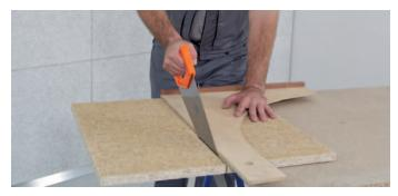
**Jack saw** – Lay the acoustic panel down with the exposed side up. Always work with a guide. Support the free end of the panel.
