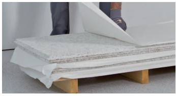
Carefully remove the separating paper layer from the panels and dispose of it immediately. Dust lying on it must not fall onto the panel below.
