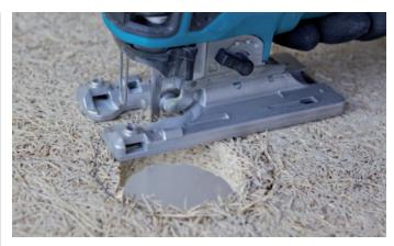
**Jigsaw** – Lay the acoustic panel down with the exposed side down. Always make longitudinal cuts with a guide.
