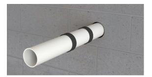
5. Push the UniWrap<sup>®</sup> into the annular gap between the wall opening and the pipe. Adjust the position of the wrap so that the edge is in line with the wall or floor surface on both sides. Seal over the top of the annular gap with FireMastic-300 in accordance with the approved system application.
