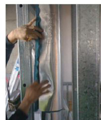
Continue lagging adjoining pipe area with the recommended overlap and joint treatment
