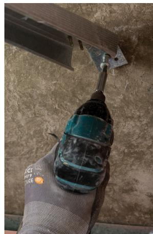
**9/** Fix GRIDLOK® top connectors to structure over with approved anchors.
