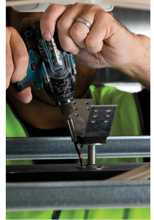
**4/** For TRACKLOK® RETRO screw directly into head track.
