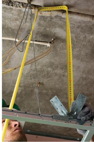
**2/** Measure distance to structure from ceiling grid.
