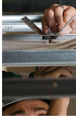
**3/** Create 9mm hole and bolt TRACKLOK® firmly to head track using washer and bolt provided.
