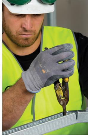
**3/** Cut your vertical steel stud to length. Will need to repeat for the two 45° steel studs as per plenum chart provided.
