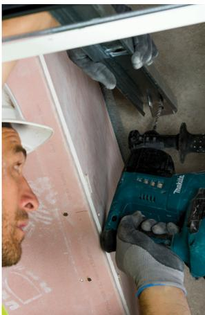
**9/** Drill clearance hole into structure over.
